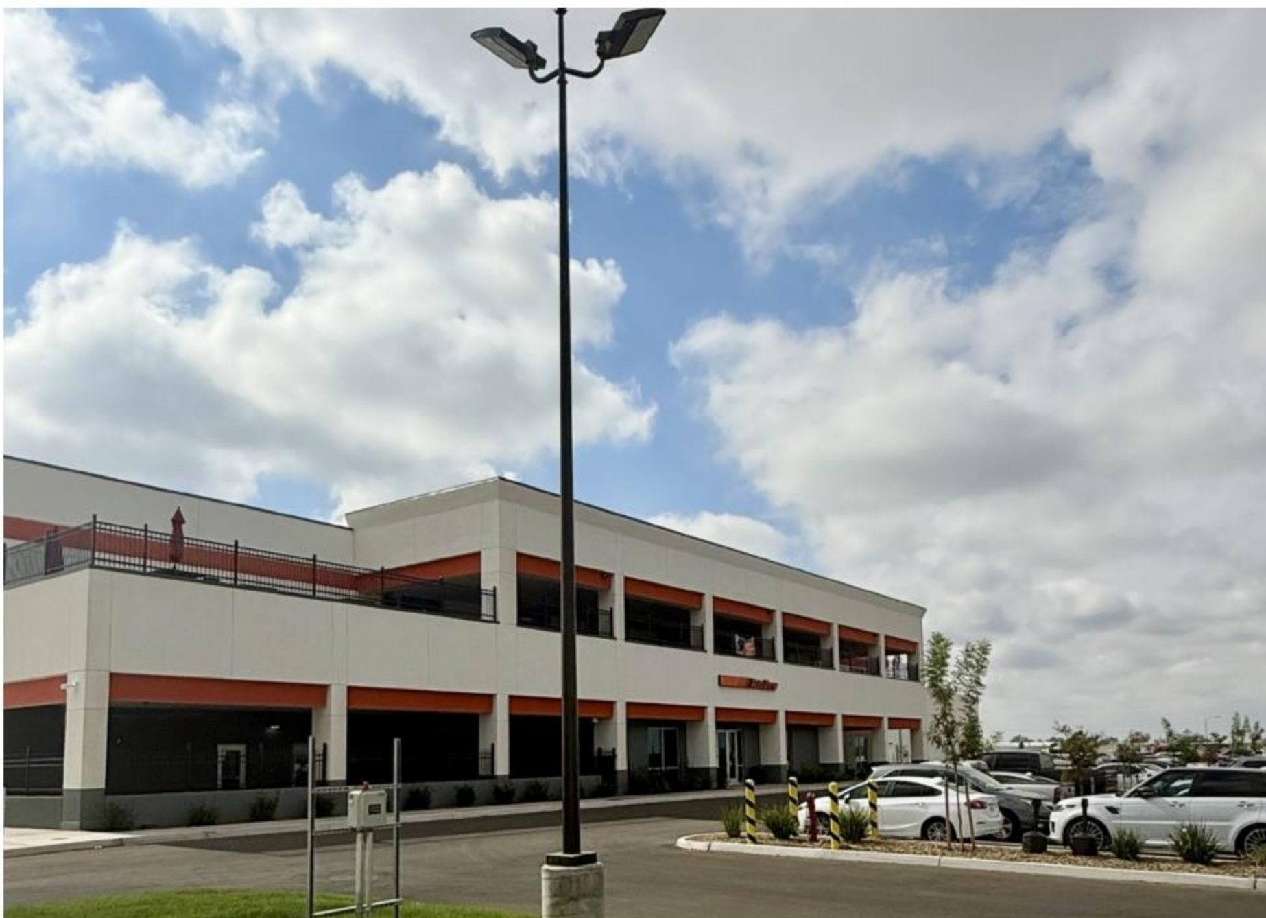
Photo courtesy of Madera County Economic Development Corporation | The AutoZone distribution center in Chowchilla put Madera County on the map for logistics and distribution investment, brokers say.
