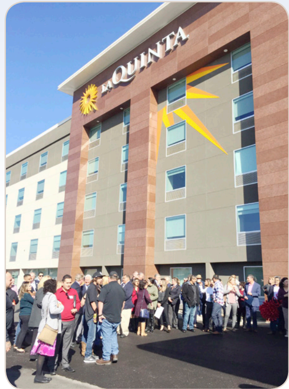
Renovated La Quinta
