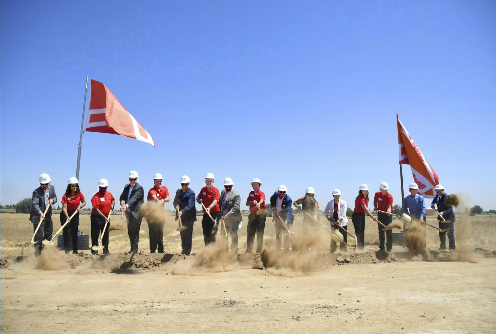
AUTO ZONE DISTRIBUTION CENTER GROUNDBREAKING
